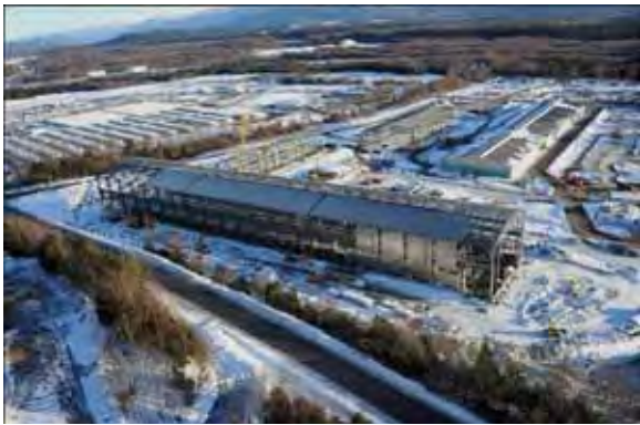
Aerial view of the Kitimat Modernization Project site. Photo courtesy of RTA/Bechtel
