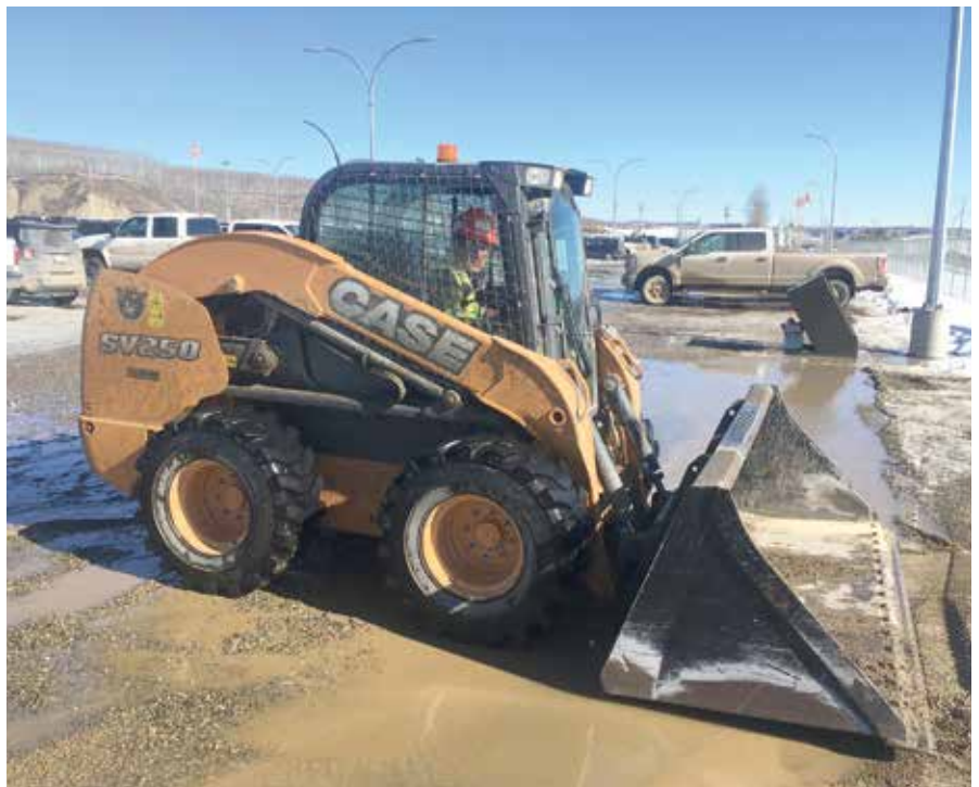
Member Ruel Maligaya on a skidsteer, working for Atco Two Rivers Camp Services Roads and Grounds, redirecting pooling water from the snowpack run off.
