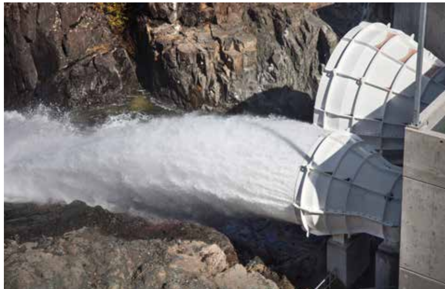
On the downstream side of the dam, the new water release valve directs water down the Elk Falls Canyon.
